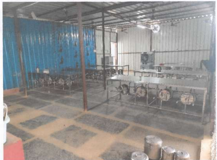
Photograph showing Kitchen & Dining hall
