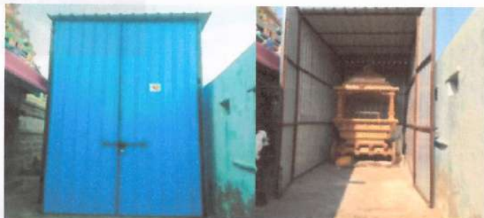
Venu Gopala Swamy Chariot shed has been constructed at Jonnagiri Village by GSMI
