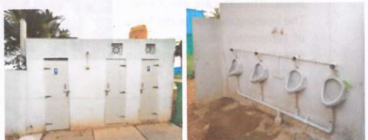
Photographs showing toilets
